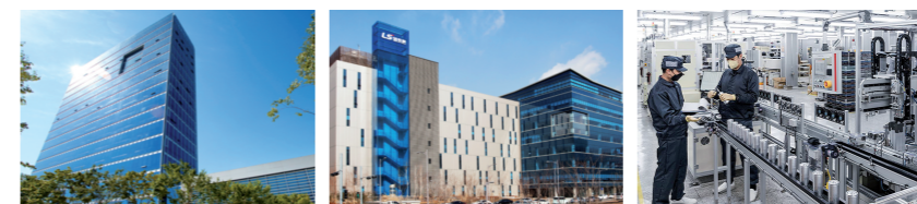
Head office, Ultracapacitor plant
